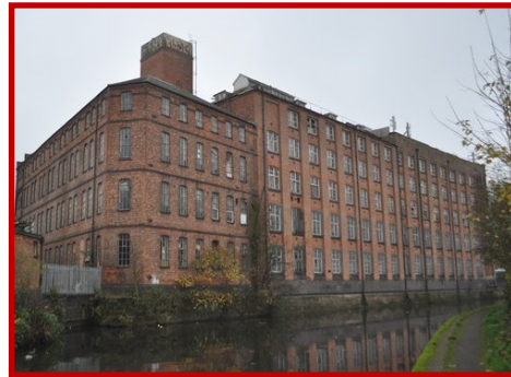
The Abbey Mills building in Leicester.
